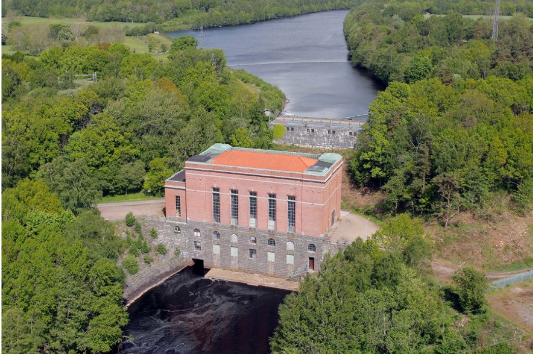
Figure 24: Karsefors hydro power plant from above (Statkraft, n.d)
